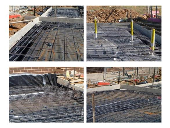
4. A number of the sewer pipes are touching the reinforcement mesh.
