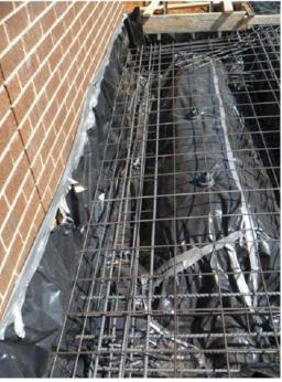
2. There are numerous areas where the reinforcement fabric is sitting on or touching the vapour barrier.
