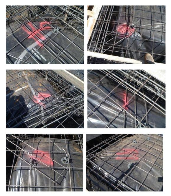
3. The biggest concern is the amount of drop in the reinforcement mesh at the perimeter and external corners of the property.
