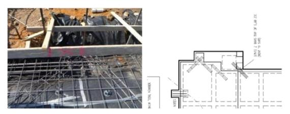
7. The sand base below the vapour barrier has collapsed into the beams in a number of areas.
