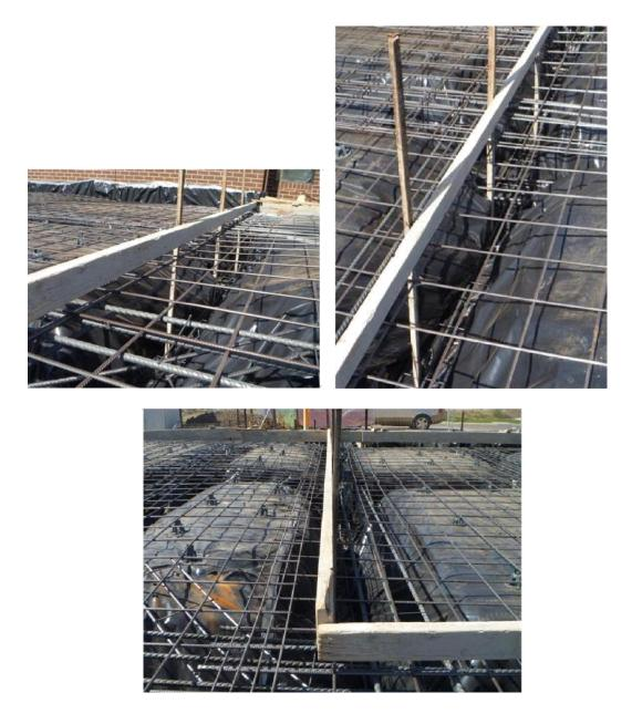
6. Front - the angled cracker bars are shown on the slab engineering to be sitting within the raised pad area.
